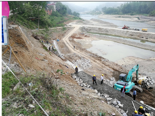
边坡拦挡及围堰
